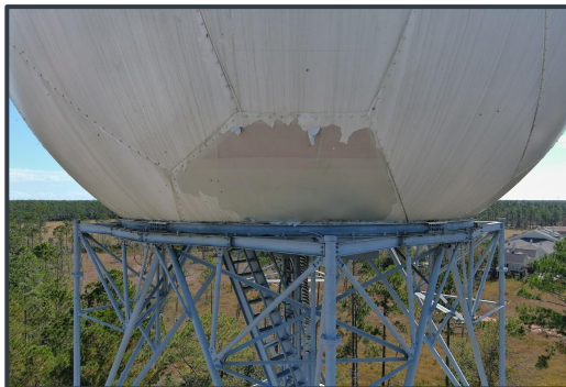
WSR-88D damaged radome panels observed from UAS
